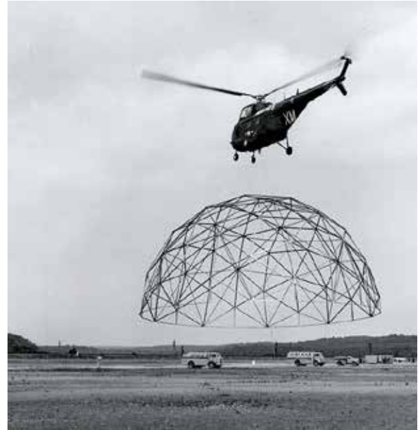
Fig. 5 - US Marine Corps transporting a 55 ft dome via helicopter, 1954. Courtesy Whitney Museum of American Art.
