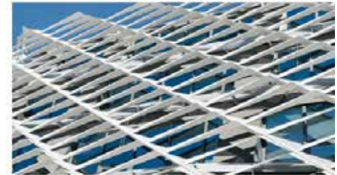
Fig. 5 - Shading devices in contemporary design, (a) Gerber Architekten, King Fahad National Library, 2015, (b) Rudy Ricciottis, MuCEM, 2013, (c) Renzo Piano, Il Sole 24 Ore Headquarters, 2004, (d) Behnisch Architekten, AGORA Pôle de recherche sur le cancer, 2018.
